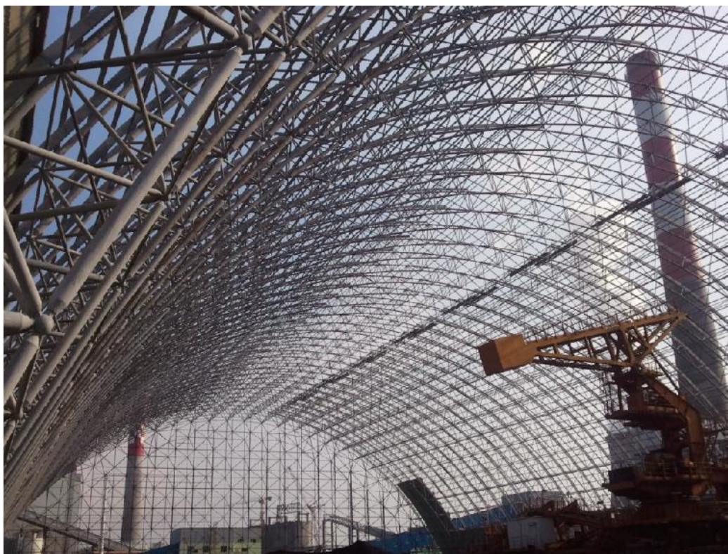
双层柱面网架结构图四
