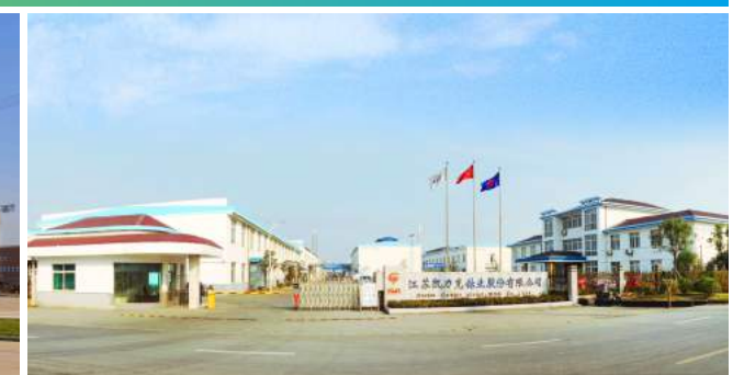
06 格林美（泰兴凯力克）电池材料产业园 GEM(Taixing KLK) Battery Materials Industrial Park
