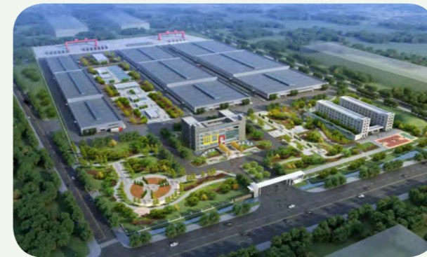
淮安循环经济产业园俯瞰图 Huaian circular economy industrial park
