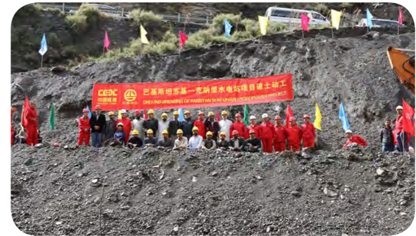
苏基克纳里水电项目破土动工 Pakistan Sue Kieker Nari hydropower project breaking ground
