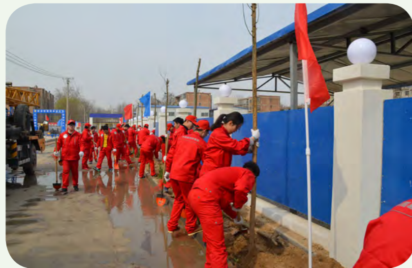
施工现场种植树木 Planting trees at the construction site
