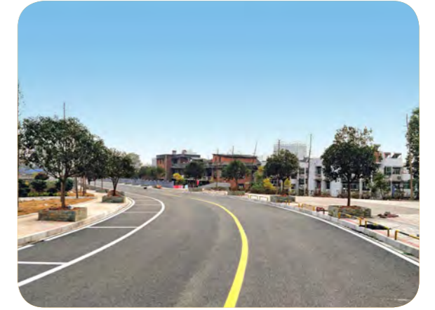
镇镜山路顺利通车 Zhenjingshan Road opened to traffic
