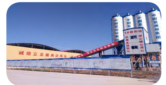
项目部安全标准化建设现场 Safety Standardization Construction Site
