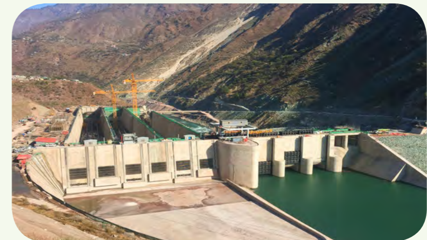
N-J 项目首部工程过水位结构全部完工图 The completed picture of N-J project first project over the water level structure
