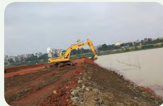
河道边坡加固 Reinforcing the river slope
