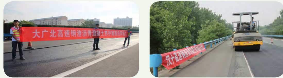
钢渣沥青混凝土技术运用到大广北、汉十高速 Steel Slag Asphalt Concrete Technology applied to Daguang North and Hanshi expressway
