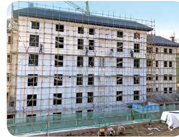
葛洲坝养老院主体工程建设 Gezhouba Nursing Home Construction Project
