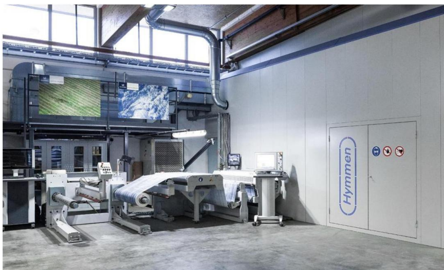
Installation of a digital printing system at the plant in Lungötz 2014
