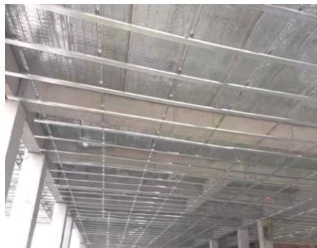
● 钢筋桁架楼承板
