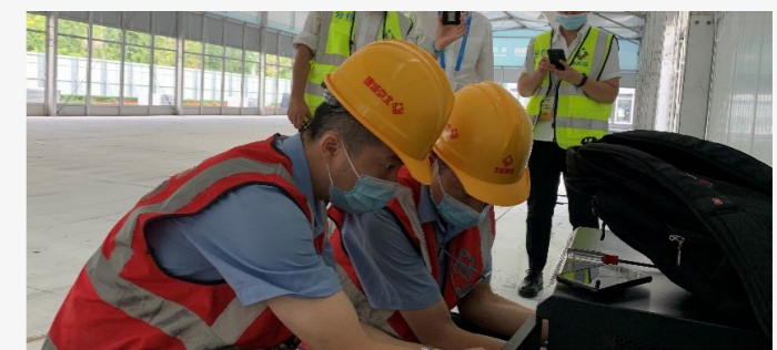
Installation and testing of outdoor equipment
