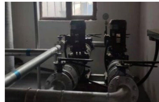
Upgrading cooling water make-up system
