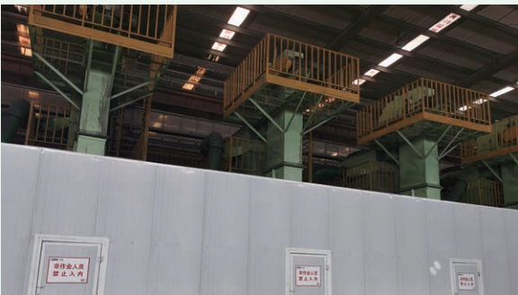
厚板线打砂机隔音墙
