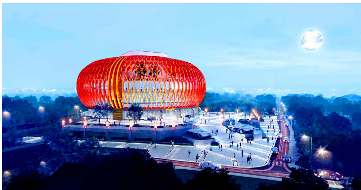
四川成都建川综合陈列馆铝合金网壳结构建设项目 Aluminium alloy reticulated shell of Comprehensive Exhibition Hall in Chengdu, Sichuan
