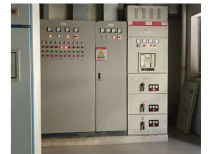
Energy-saving transformation of central air conditioning
