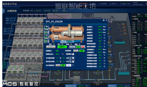
Operation Screen of Water Chiller
