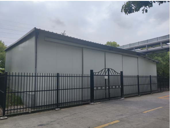
Wastewater treatment pool
