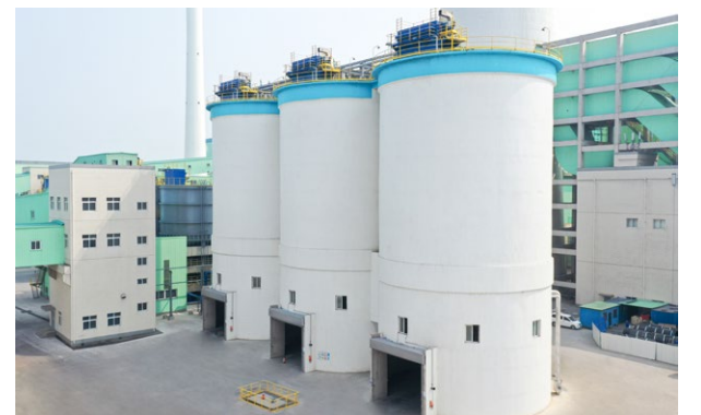
Hengli Petrochemical Refining fly ash recycling system
