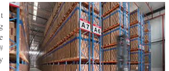
Warehouse expansion and renovation
