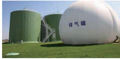
Biogas power generation system
