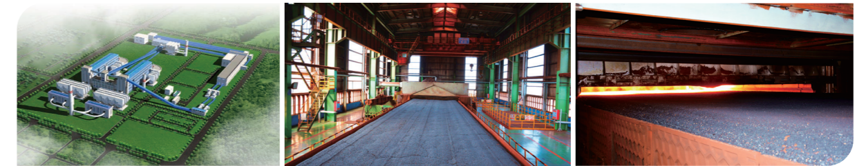
Sintering reuse system
