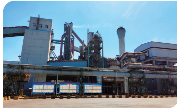
Ground granulated BF slag production line
