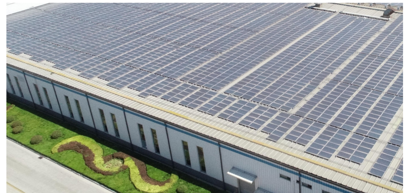
CTG's Photovoltaic Project
