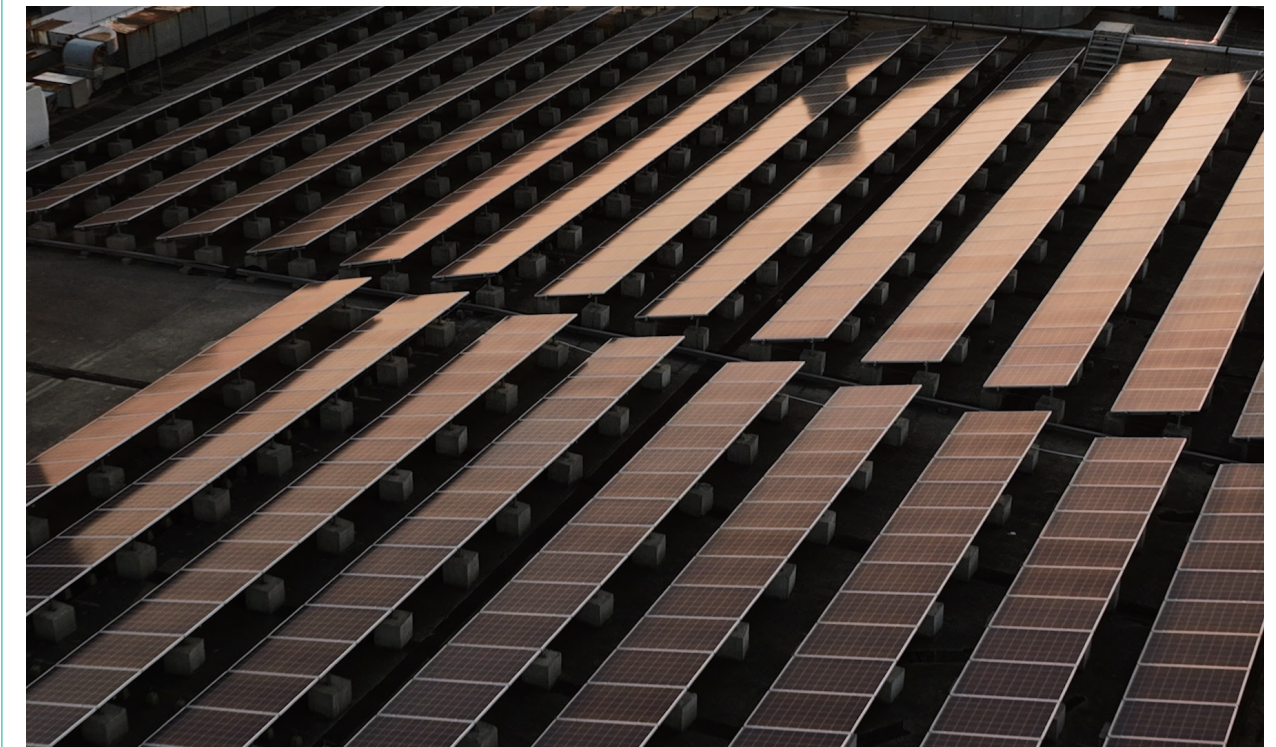
Installation of the distributed PV
