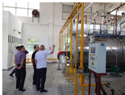
Safety Inspection for the Second Quarter
