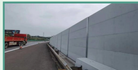
Site picture after sound barrier installation
