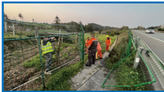
Demolition of illegal roadside structures
