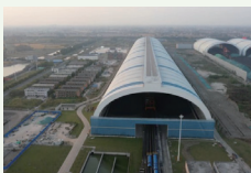
封闭式干煤棚
