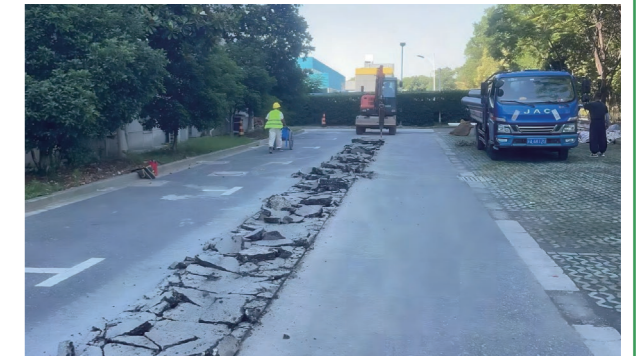
Pipeline laying
