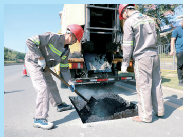
● “四新”技术试验现场
