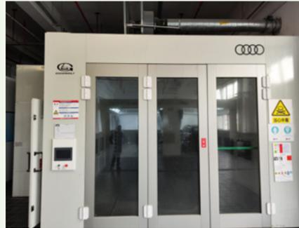
we have installed standard-compliant VOCs equipment for filtration and regularly replaces the equipment's filter elements. Our VOCs exhaust gas treatment process is suitable for medium-concentration pollutants, with workshop spray exhaust gases being drawn into the XHTML VOCs purification device by an air delivery system. The equipment consists of a primary filter, flat plate filter, and adsorption sections. Dry filtration is used to remove paint slag, with fine particles in the exhaust gas
