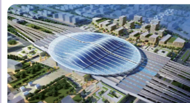
Xiongan New Area High-speed Railway Station Project
