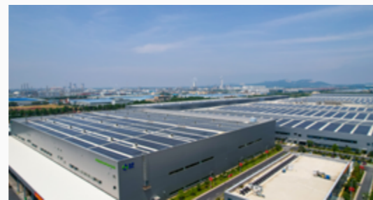
Hefei GCL SI Xinyu PV Power Station
