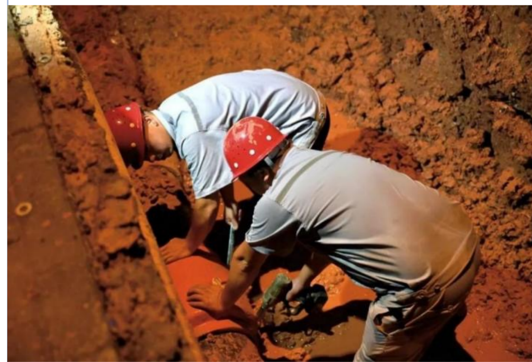
Water supply infrastructure construction
