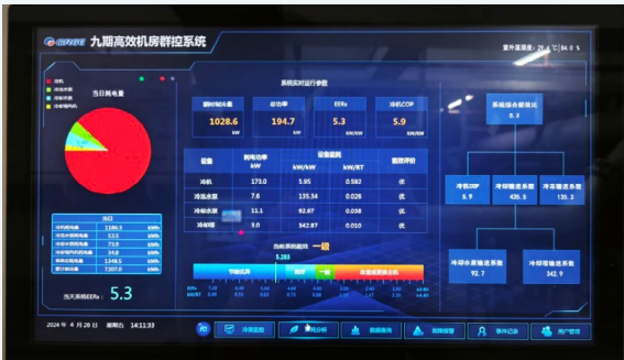
Improving energy efficiency in the air conditioning machine room of Zhuhai headquarters
