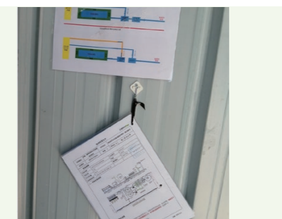
Sewage treatment station after rectification (with the Safety Operation Procedures posted)
