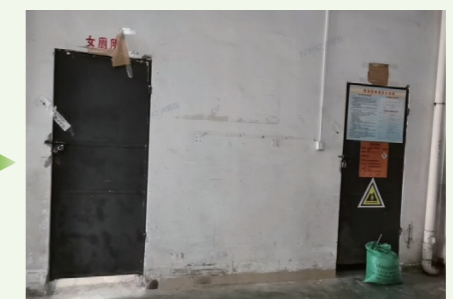
Hazardous waste warehouses after rectification (with debris removed)
