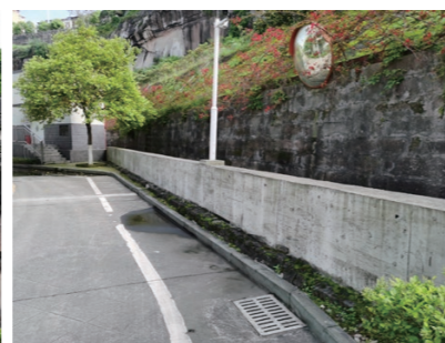
Prevent Flood Inundation - Raise the drainage channel
