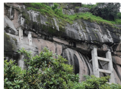
Prevent Landslides - Reinforce the slope of the rear mountain
