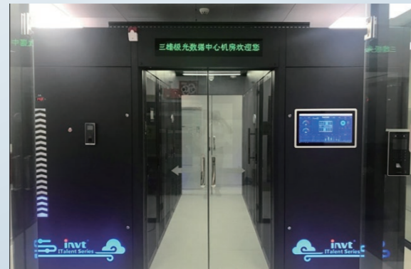
Data Collection Platform Server of PAK
