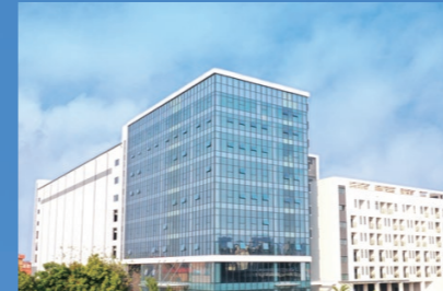
Nansha LED Smart Lighting Production Base
