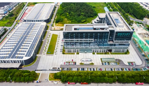
Estun Automation Headquarters Robot Manufacturing Base
