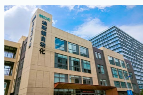
Central China Regional Headquarters (Changsha)
