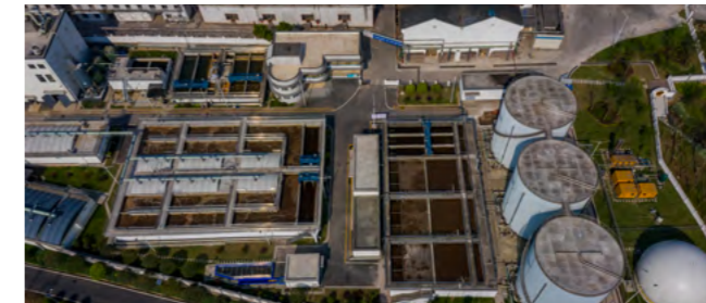
Wastewater Treatment Station in Luohan Brewing Ecological Park
