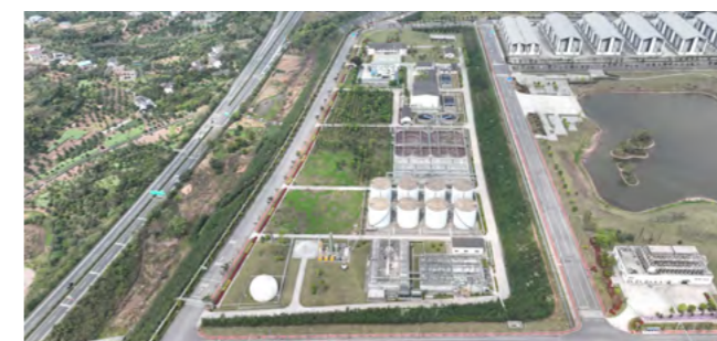
Wastewater Treatment Station of Huangyi Brewing Ecological Park
