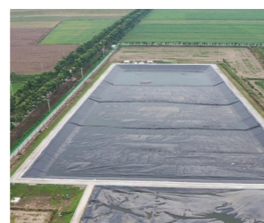
Black membrane anaerobic lagoon
