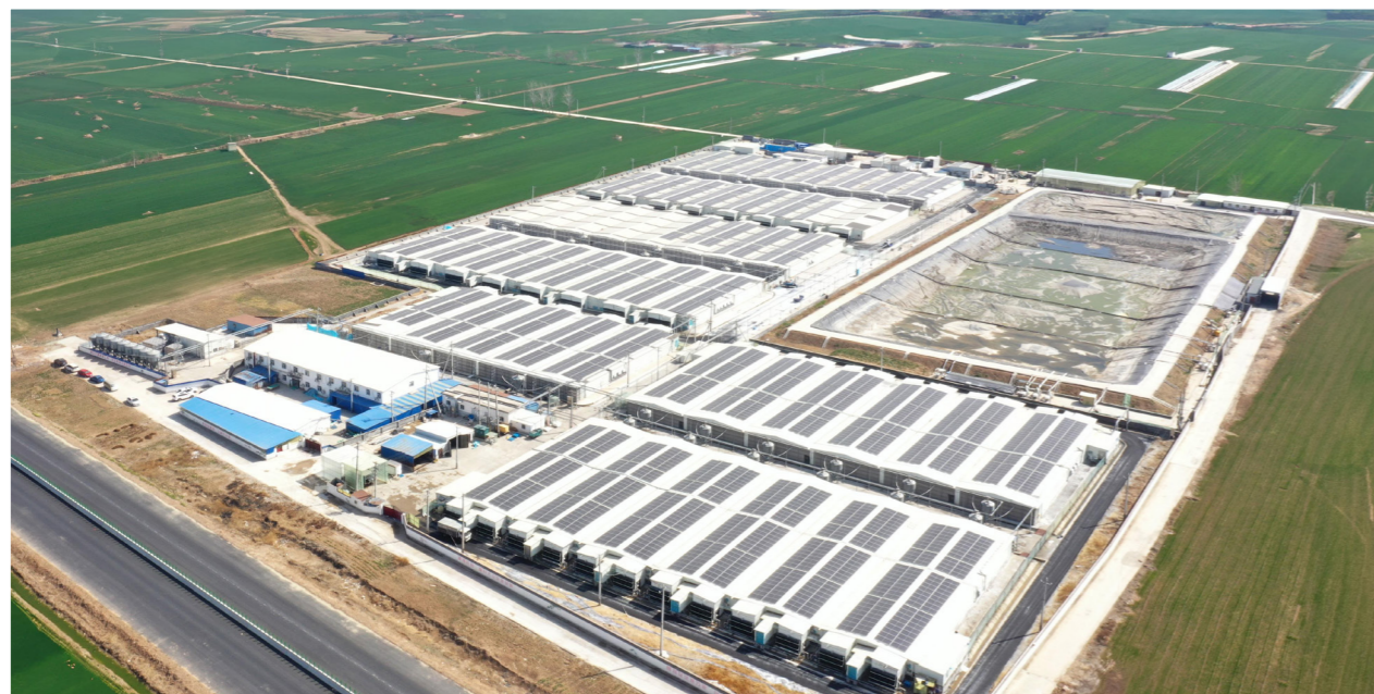
Aerial View of the Photovoltaic Power Generation Project in Suiyang Farm No. 5, Henan
