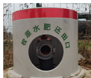
Biogas slurry land application facilities
