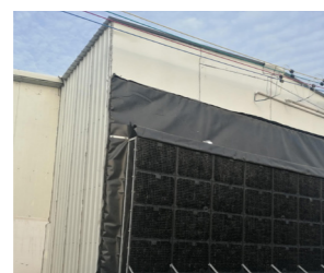
Solid-liquid separation facilities
