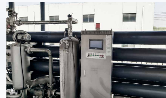
Steam waste heat recovery facilities
