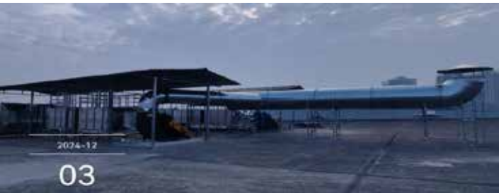
Wave soldering and three-proofing coating waste gas treatment facilities
