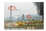
Infrared over-height detection device
