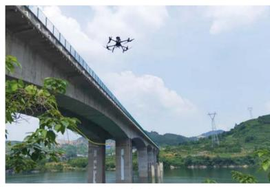
Huaihua Branch uses DJI drones for highway maintenance inspections.
