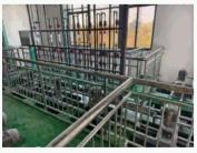
Water Reuse System of Anodizing Wastewater Treatment Stations, with a 60% Reuse Rate
