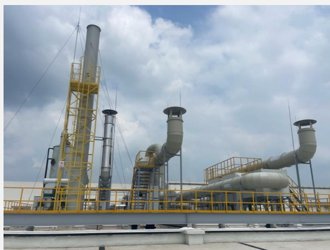
Waste gas treatment device
