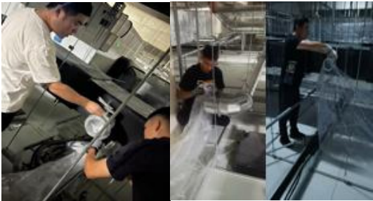
▲ Sealing of Reserved Ventilation Openings
