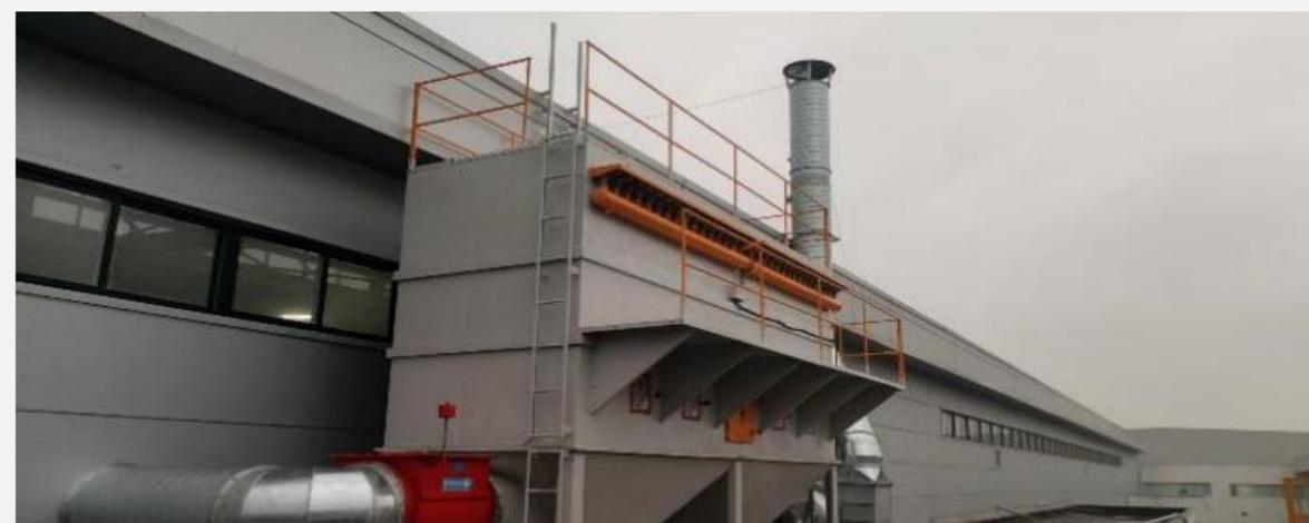
• New high-efficiency pulse bag dust collector
