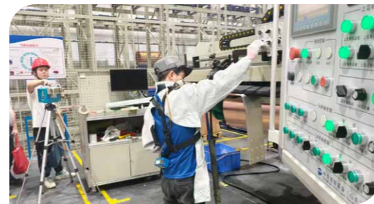
Environmental inspection at the construction site
