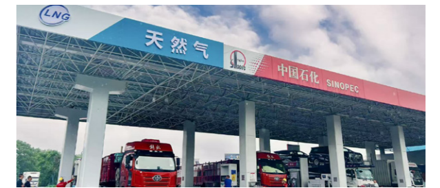
LNG Refueling Station at Shaoshan Service Area
