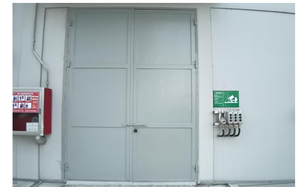
General Solid Waste Warehouse
