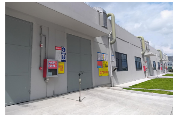
Hazardous Waste Warehouse
