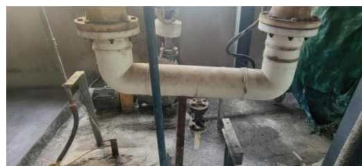
Replace the drain valve at the U-bend of the gas phase pipe of the solid mother liquor kettle with a double valve.
