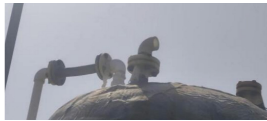
The pp elbow connected to the soft connection at the flange of the y metering tank v1006 on the third floor of jiacha was replaced due to leaks.
