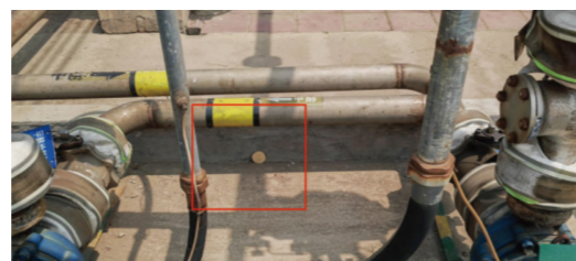
Change the anti-spill containment for pumps in the raw material area to wooden drain plugs.
