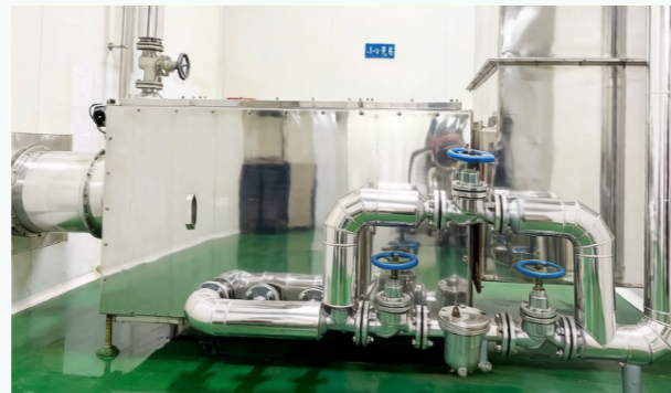
Upgrading and renovation of the fluid bed dryer heater
