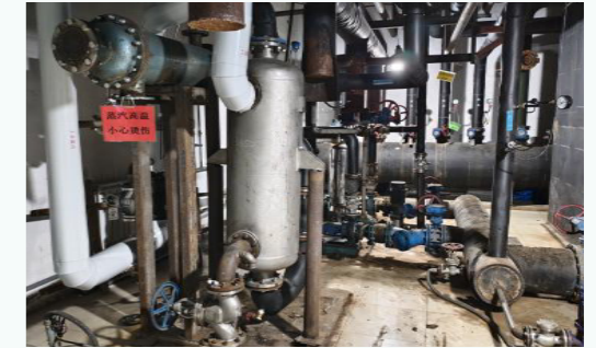
Addition of an automatic control system for the heat exchange station
