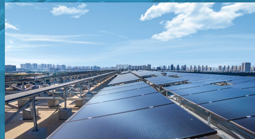
2.2 MW of Photovoltaic Capacity
