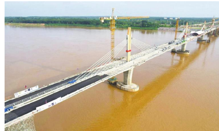
Construction Site of Fifth Lao-Thai Friendship Bridge
