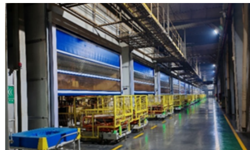
Environmental Protection Facilities at Hubei Linglong
