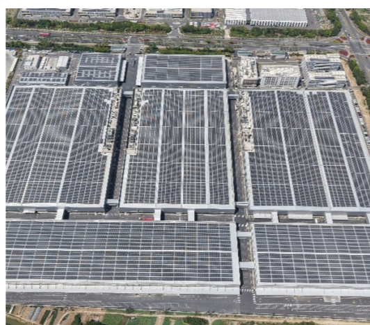
35 MW Distributed Photovoltaic Project of HY Solar (Wuxi)
