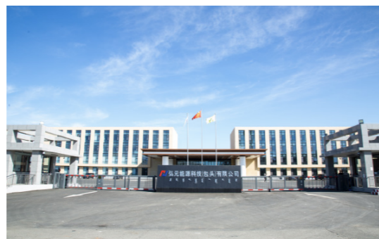
Hongyuan Energy (Baotou) Energy Production Base
