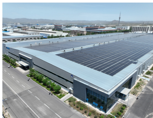
Photovoltaic Project of Hongyuan New Material (Baotou)
