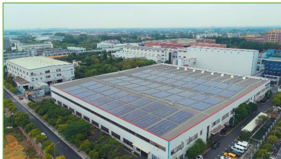
Figure: Self-built Rooftop PV Power Station Project
