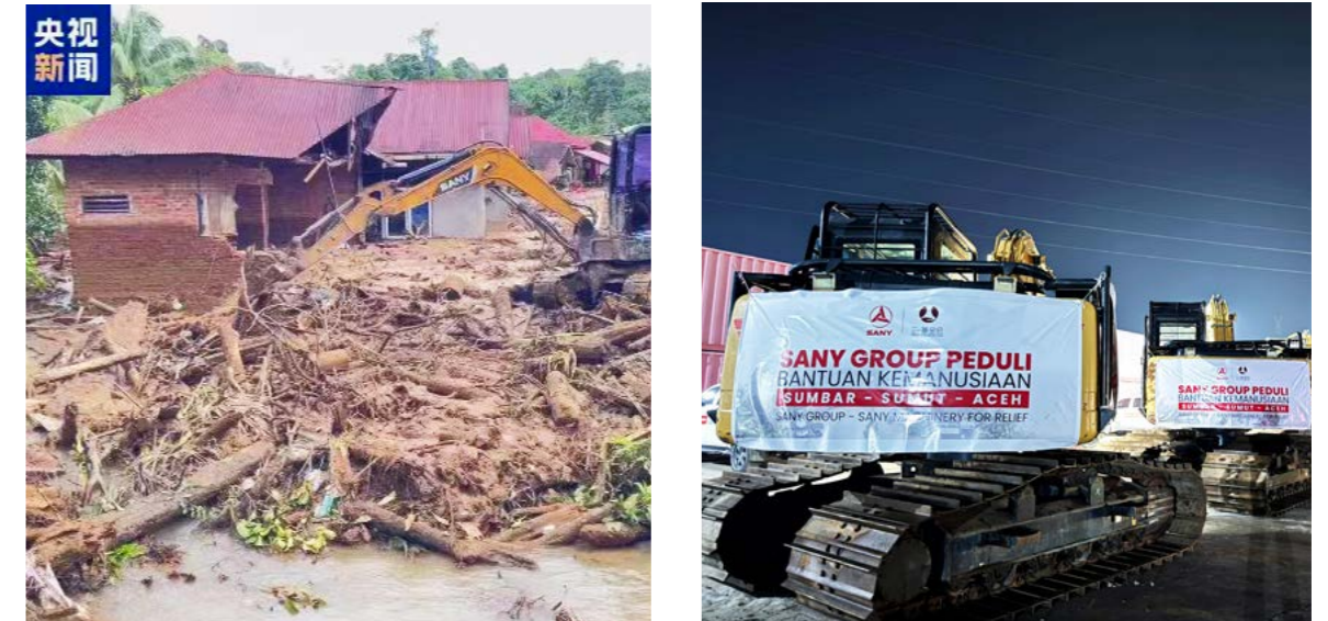
SANY Heavy Industry's Flood Relief Operations in Indonesia
