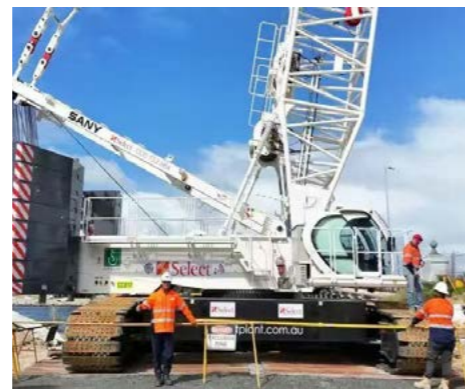
SCC3200T Crawler Cranes in the Fremantle Bridge Renovation Project in Australia
