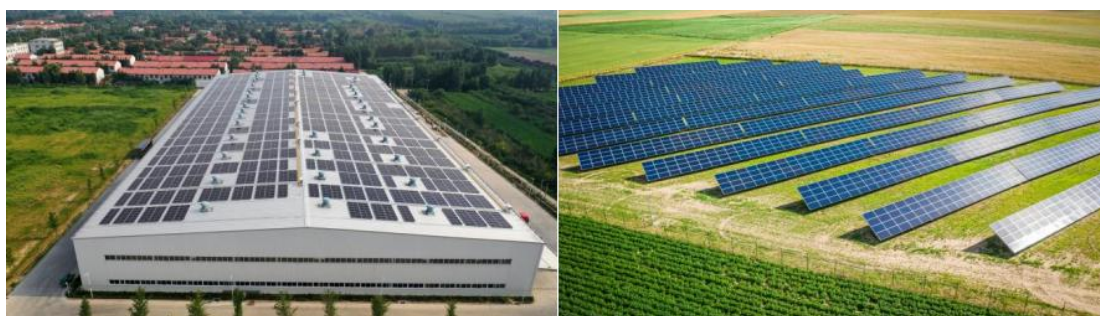
Figure: Hengyi Brunei Natural and Renewable Energy Sustainable Integration Project
