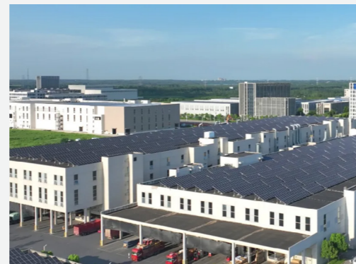
Photovoltaic Power Station
